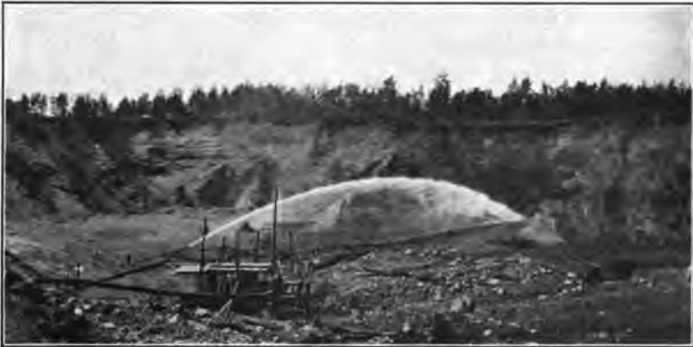
HYDRAULIC METHOD OF STRIPPING OVERBURDEN
